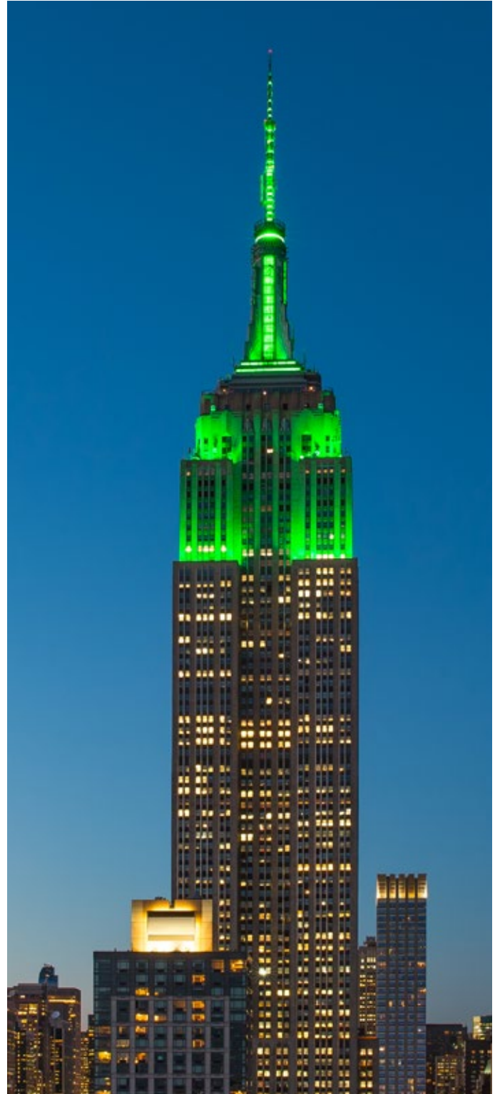
Empire State Building illuminated in Garden green
