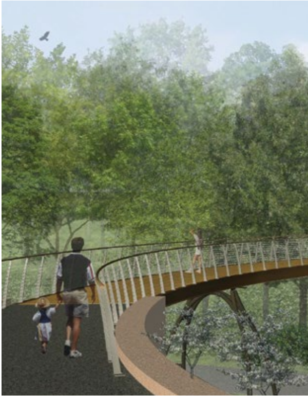
The new East Gate's pedestrian bridge
